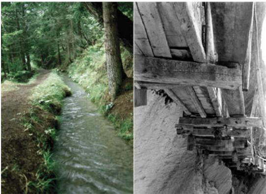
Figure 2: Channel Cut into the Valley Side, the Bisse of Ayent (Left), and Wood Channel, the Former Bisse of Savièse (Right)
